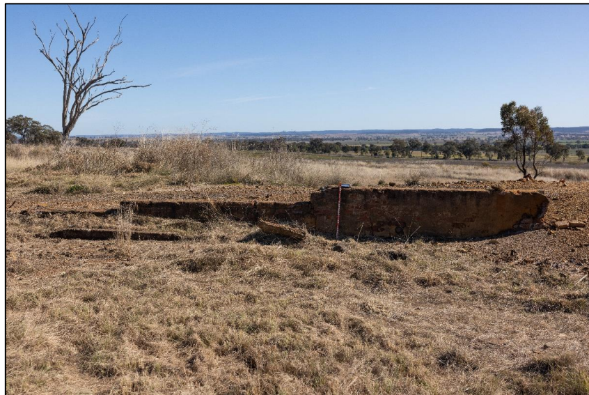
Figure 3-2: LV 14 retaining wall facing west (Everick Heritage 2022)
