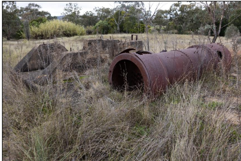
Figure 3-10: LV 29 view of the boiler footings, and metal boiler structure located adjacent to the original footing location (Everick Heritage 2022)
