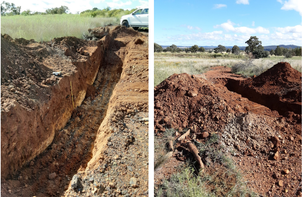
Figure 8 Backfilled contaminated material in areas devoid of vegetation (Mt Stewart Drainage)
