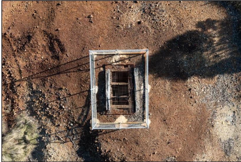
Figure 3-9: LV 28 drone picture showing the previous remediation works (Everick Heritage 2022)
