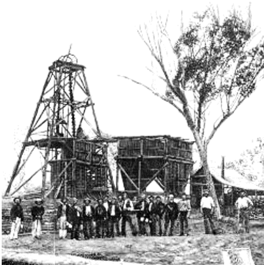
Figure 2-7: Etching showing the poppet head and hoppers at Leadville Mine (Source: Sydney Mail, 27 August 1892; via Trove)
