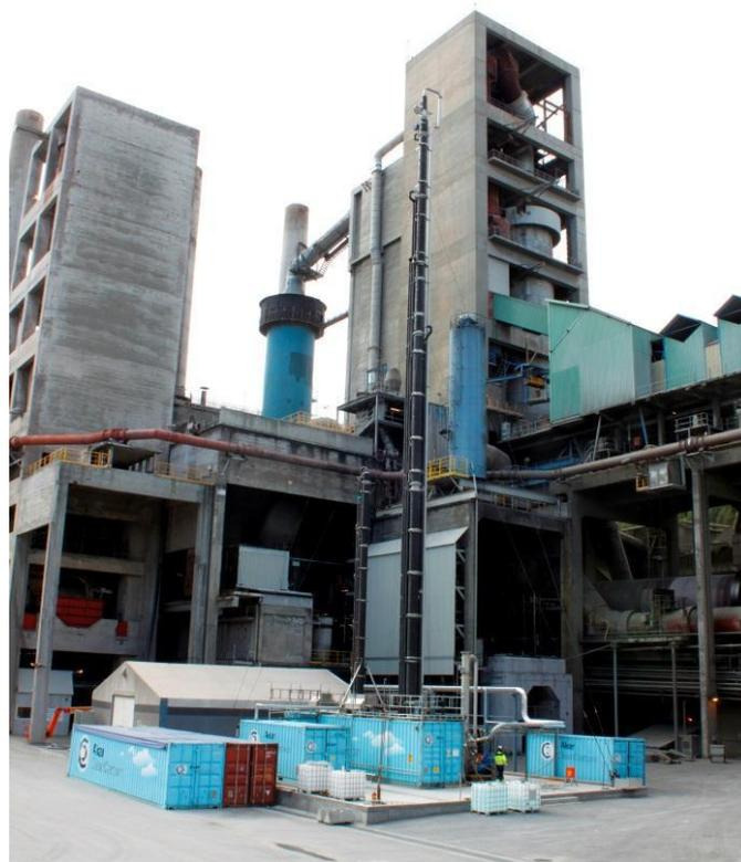
**Figure 4: The Aker Solution's MTU installed at Norcem's cement plant<sup>39</sup>**
