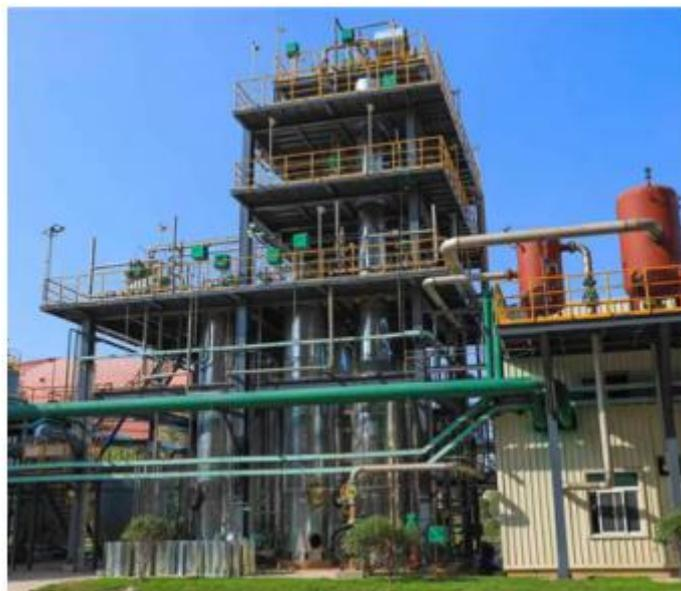
**Figure 5: The 50,000 tpa amine-based CO<sub>2</sub> capture plant in China<sup>31</sup>**
